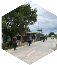
CONCRETE ROAD, COMPLETED
