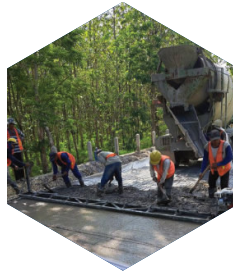
RIGID PAVEMENT WORKS
